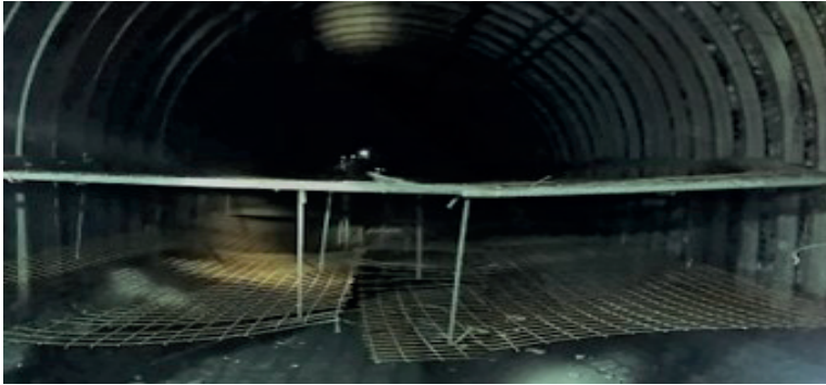
Figure 2- Reinforcement of the artificial ceiling
