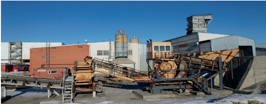
Figure 4. Concrete backfilling plant of the Pervomayskiy deposit
