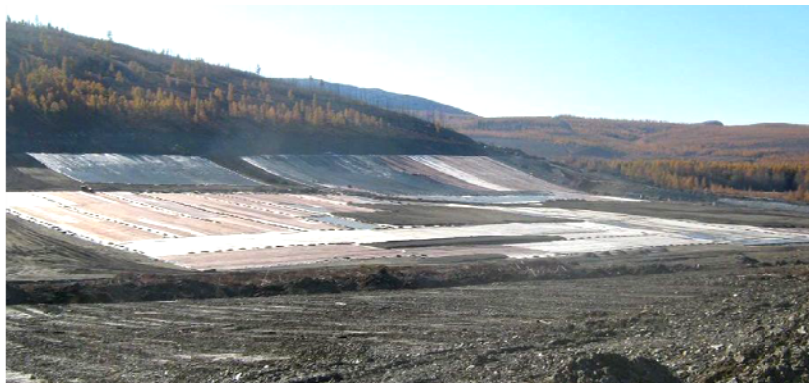
Figure 1 – The Use of Geosynthetic Screens in the Development of industrial waste storage
