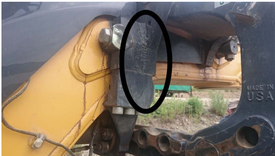
Figure 16 – Welded crack on the mounting bracket of the grader hydraulic rams, caused by unaccounted real loads
